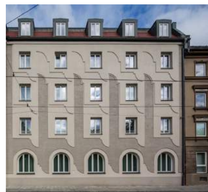
Munich. Housing block renovation.
