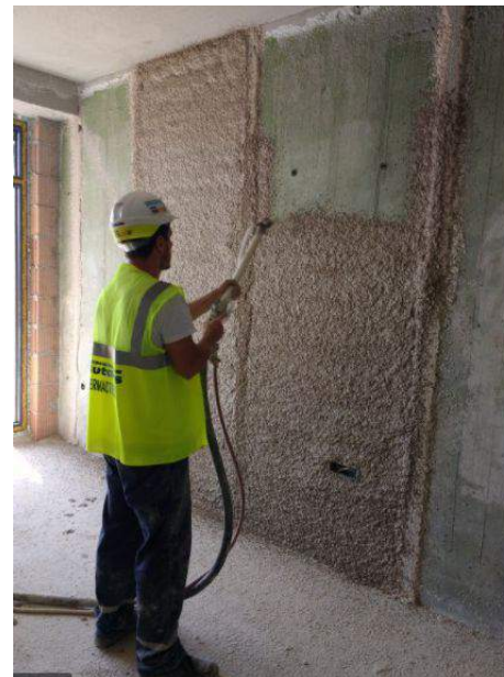
Wet applied insulating plaster
