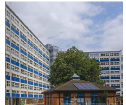
Wilmcote House, Plymouth City Council
